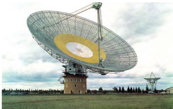
In 1970, the inner 33 metres of the dish surface were replaced by perforated aluminium panels. They appear yellow in this picture but were later painted white to reflect the heat in order to minimise the surface deformation. The panels were later progressively extended to 37 metres, then 45 metres and finally to 55 metres in 2003. Image Copyright: CSIRO
