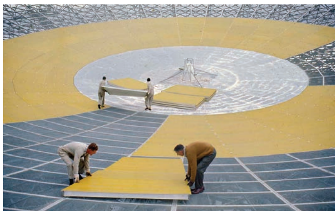
In September 1970, the Parkes Observatory director, John Bolton, is seen on the right installing the first of the new aluminium panels, with his staff. Image Copyright: CSIRO
