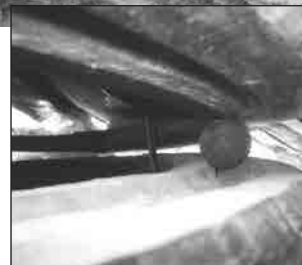
The Dawes Observatory was built onto the side of a rocky outcrop to help stabilise the instruments. The observatory dome was a wooden frame with canvas. It ran on a track with cannon balls. This reproduction can be found at Old Sydney Town (near Gosford, NSW)
